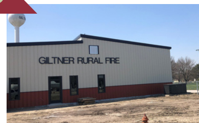
Giltner Fire Department new fire house
